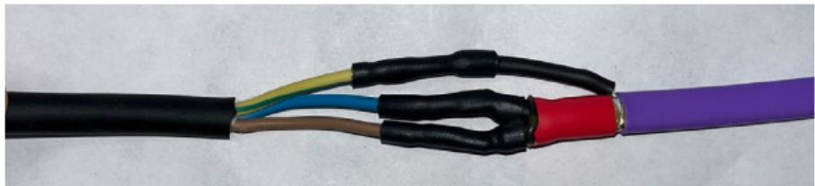
Center the shrink tubing 19/6x130mm over the connections and heat from the center and outwards
