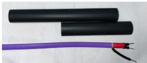
Install shrink tubing 8/2x35mm over the 3 wires on supply cable and crimp on the ferrules
